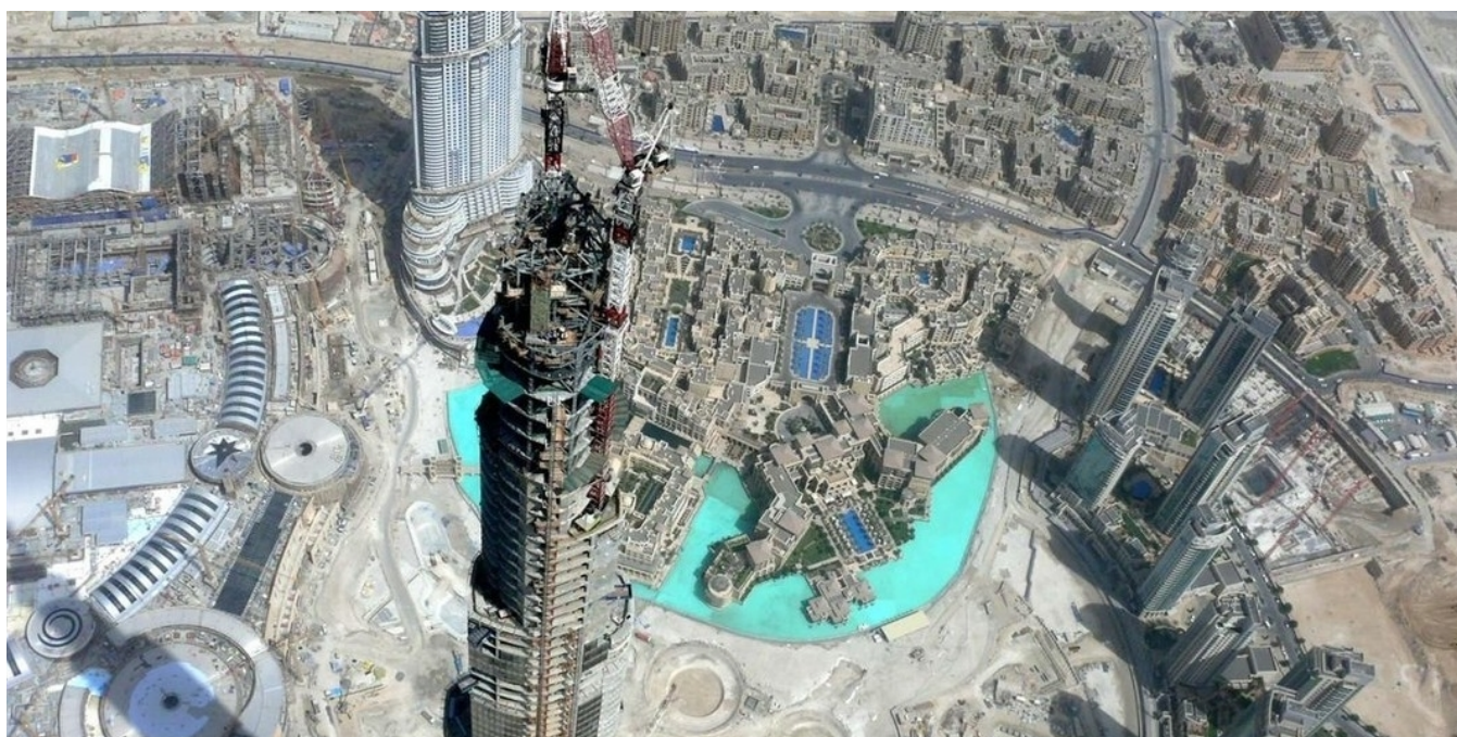
The Burj Khalifa under construction in Dubai, 2008. Photo: Imre Solt.
