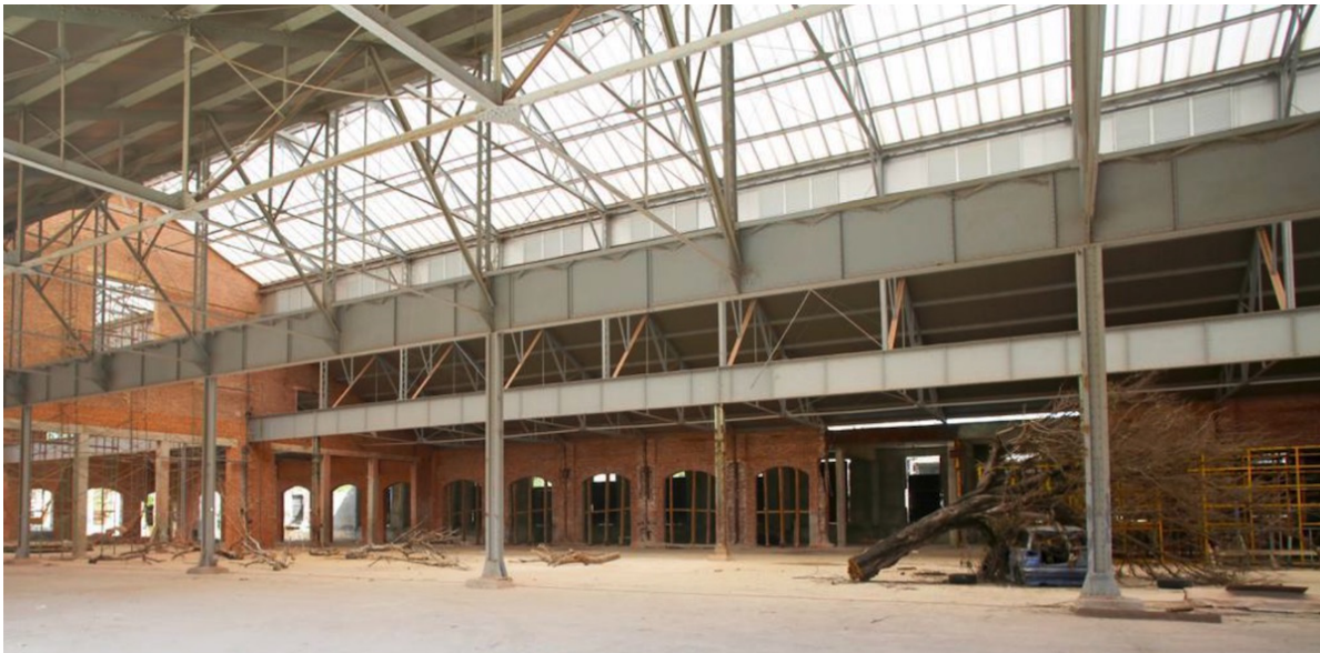
Installation view of Glenda León's "Mecánica Natural / Natural Mechanics," 2019, in Nave Línea y 18 Courtesy Estudio Glenda León
